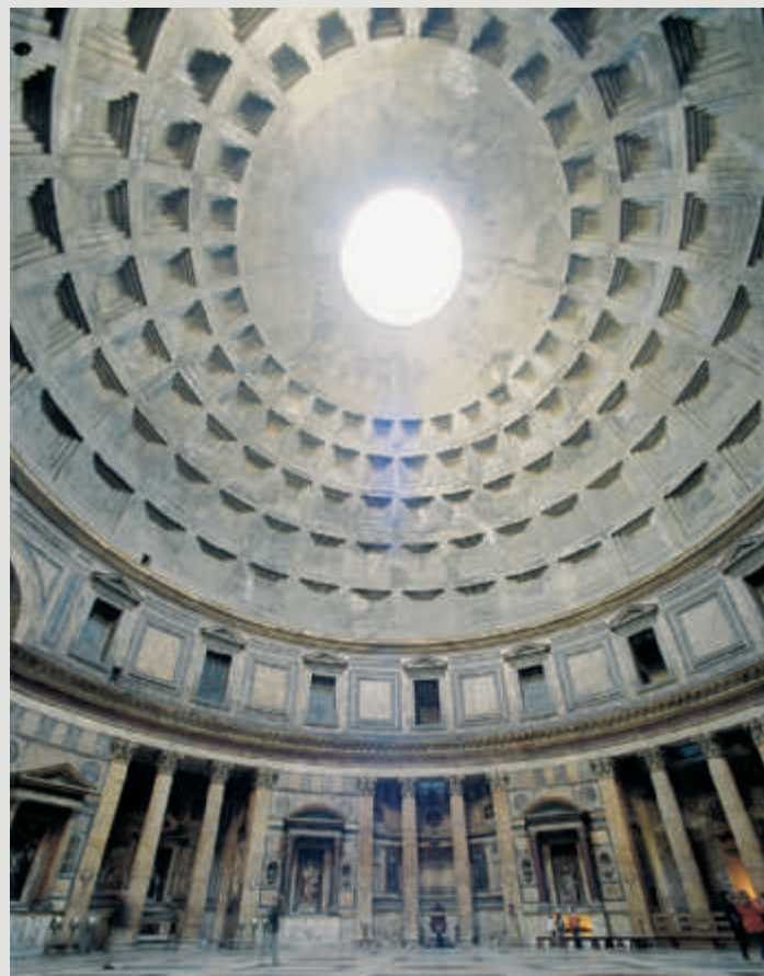
Roman dome with oculus (Pantheon, Rome, Italy, 118–125)
